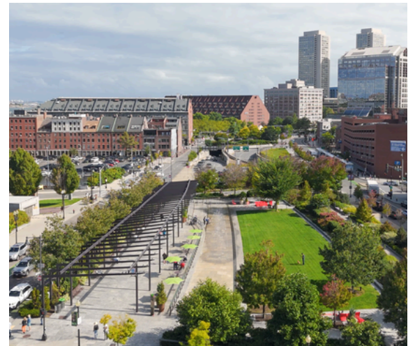
North End pergola and fountains
