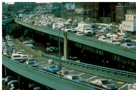
The elevated highway that once occupied the space where The Greenway lives today in the North End
